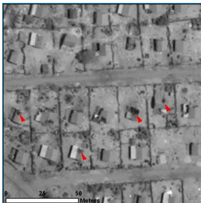
By May 10, 2009, other structures had sustained damage (indicated by red arrows). Image © 2009 DigitalGlobe
