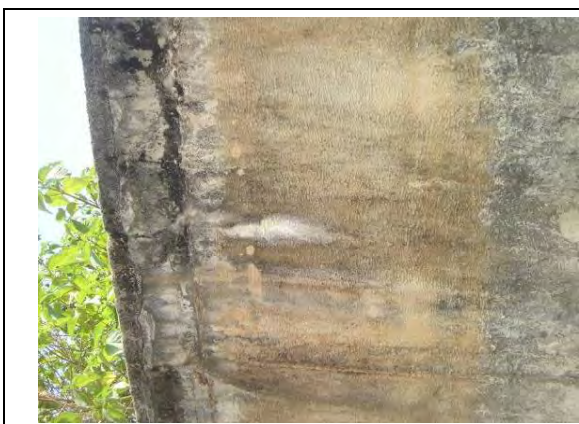
Slow Sand Filter (Internal Wall)
