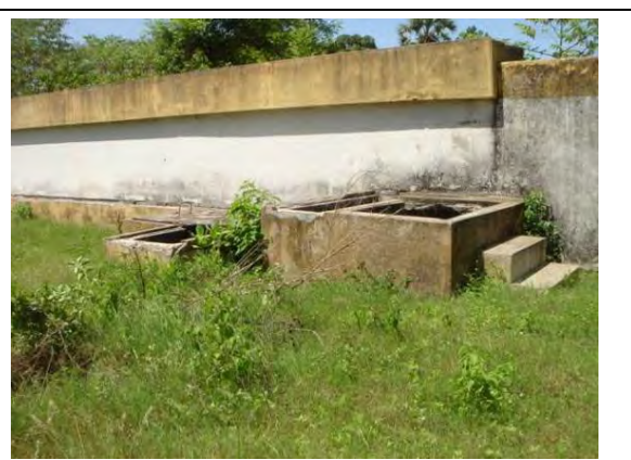
Slow Sand Filter (External Wall)
