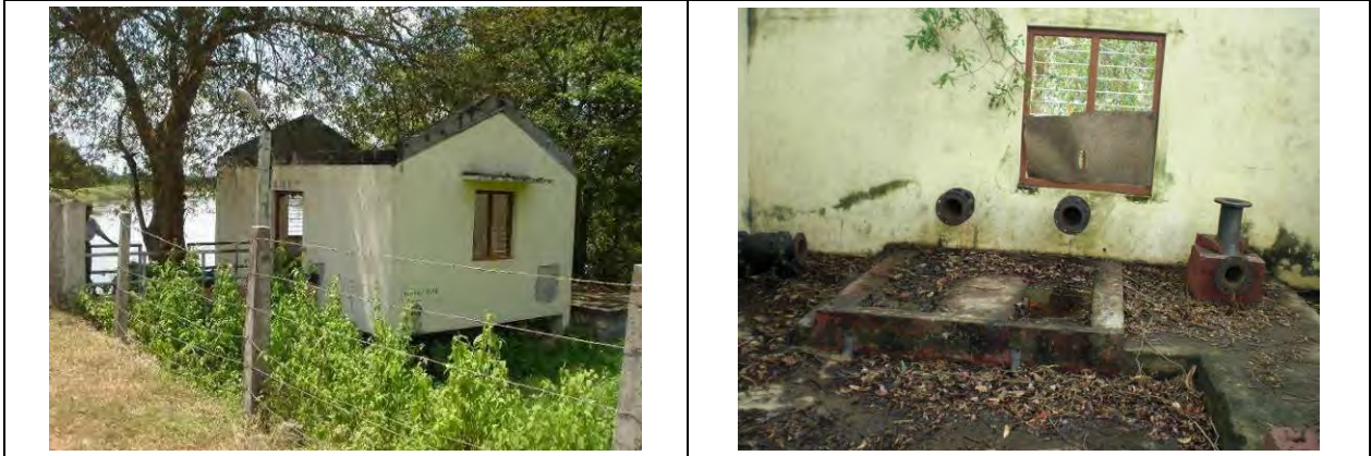
Intake Pump House (Outsied)
