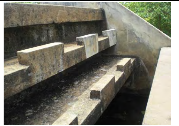
Existing Aerator (Cascade)
