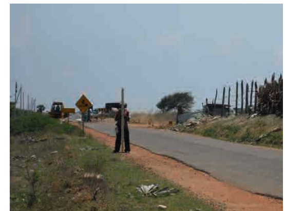
Photo Control Point Survey(Leveling)
