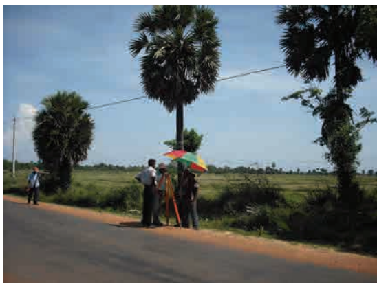
Photo Control Point Survey(Leveling)
