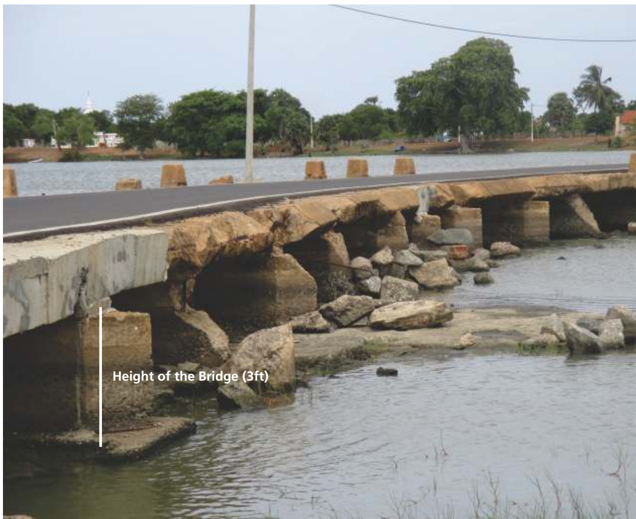
Poor condition of Vadduvakal Bridge
