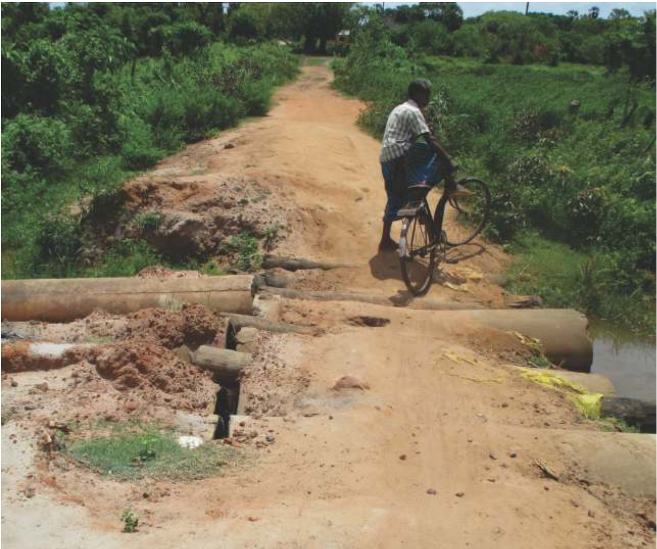
Interior road in Mulliyawalai with dilapidated culverts
