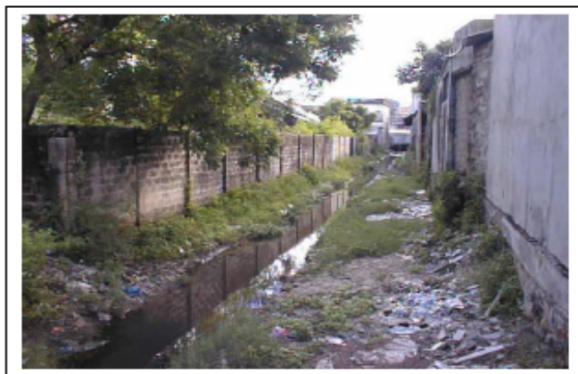
Plate 3.2.12: Waste Water Flow in Storm Water Outfall Channel
