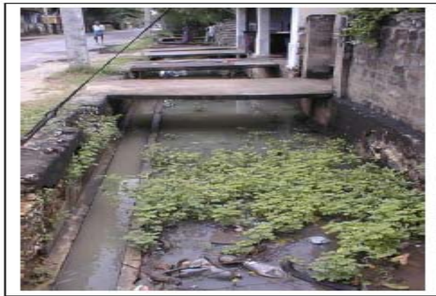
Plate 3.2.13: Large Storm Water Drain with integrated Waste Water Channel
