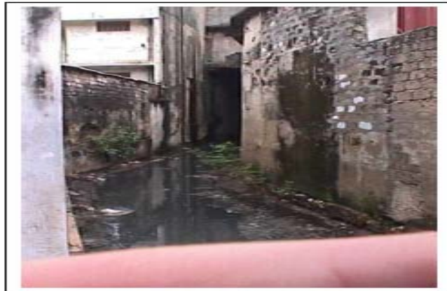
Plate 3.2.11: Waste Water Flow in Storm Water Channel in City Center
