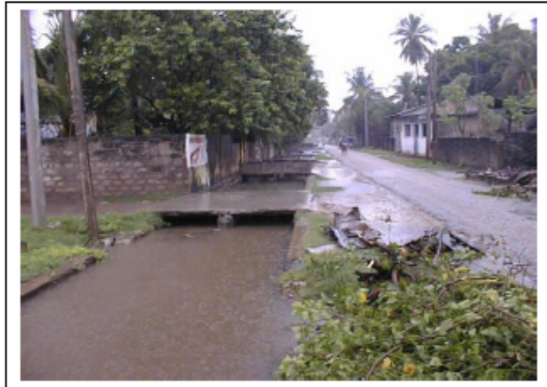
Plate 3.2.10: Storm Water Channel under full load
