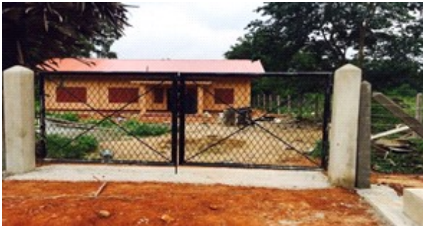
Construction of a Multi-purpose hall
