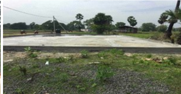
Construction of a Paddy Drying Platform
