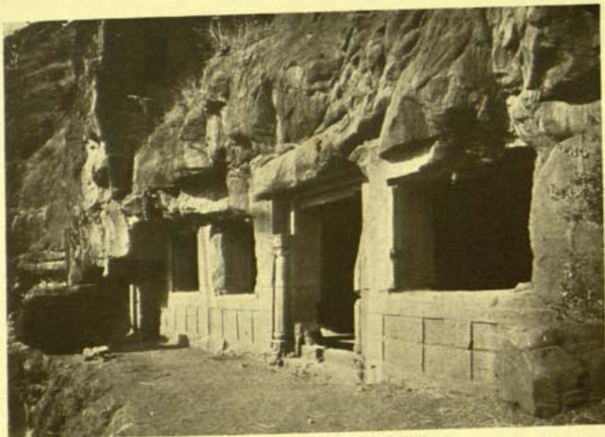
FAÇADE OF THE LOWER STOREY. CAVE 6.
