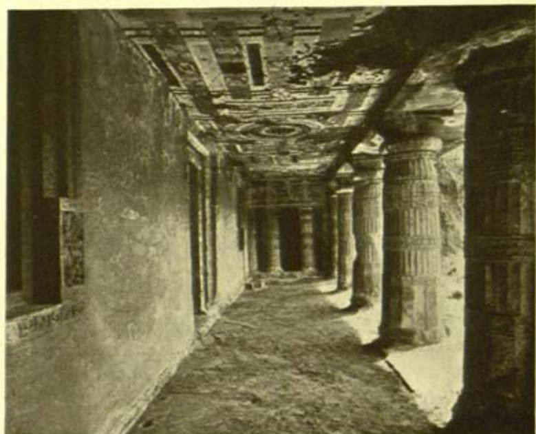
CEILING OF BARANDA.
