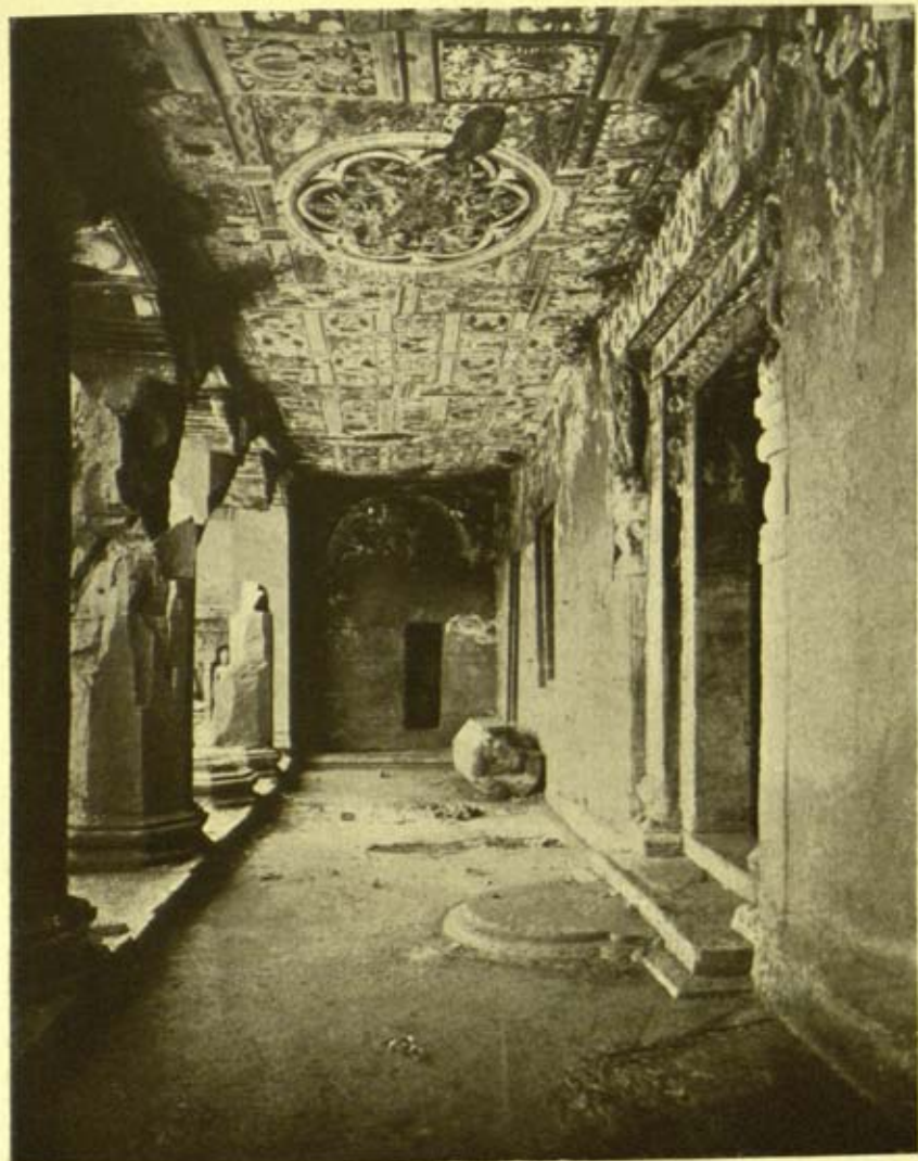
CEILING OF BARANDA. CAVE 17.
