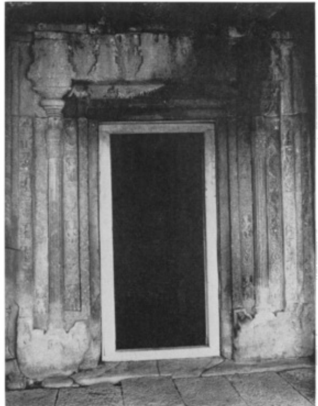
FIG. 53.—Aihole. Two-storied Jaina Cave. Outer door frame of lower story (Tarr 170, 20).
