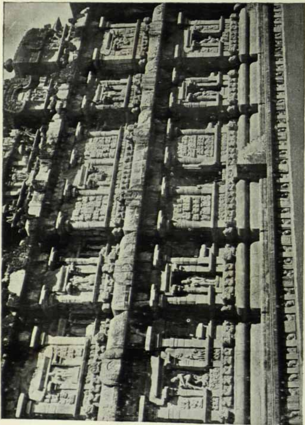
4. South wall of the vimāna
