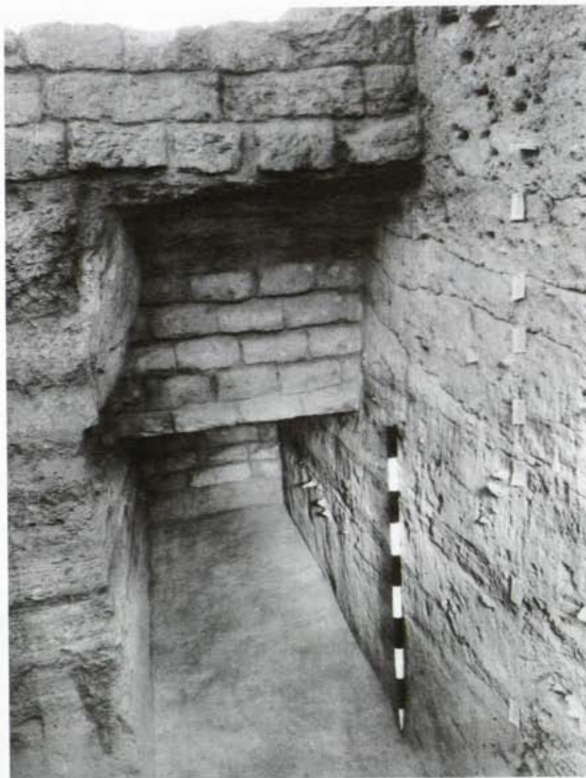
Pl. VIII KLB-1: Early Harappan defence wall of two phases and Harappan revetment. See pp. 21&52
