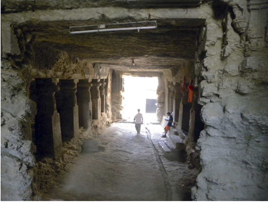
FIGURE 73 Approach to Jogeśvarī caves
