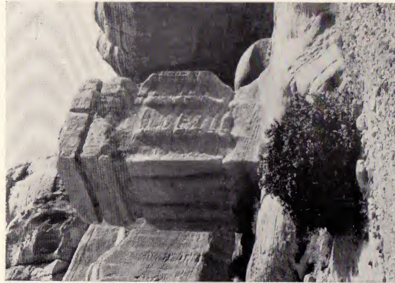
Fig. 2. Recent Photographs of 'Sahrij' Monument in Bab el Siq. Note clear indication of Hegrtyp architectural ornament with chases cut in natural rock for inseting cornices etc. in different stones.
