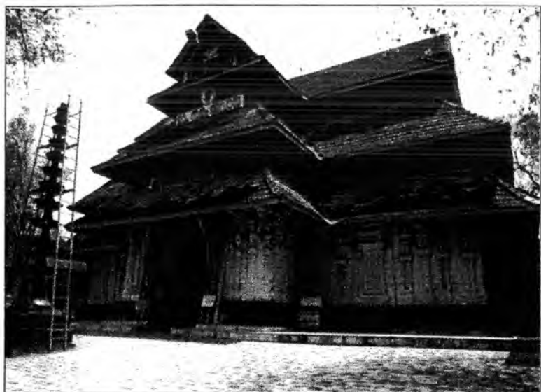
GŌPURA - TYPICAL KĒRAḶA STYLE (Western (front) gōpura of Śree Vatakkunaathan temple, Thriśśūr, Thriśśūr district)
