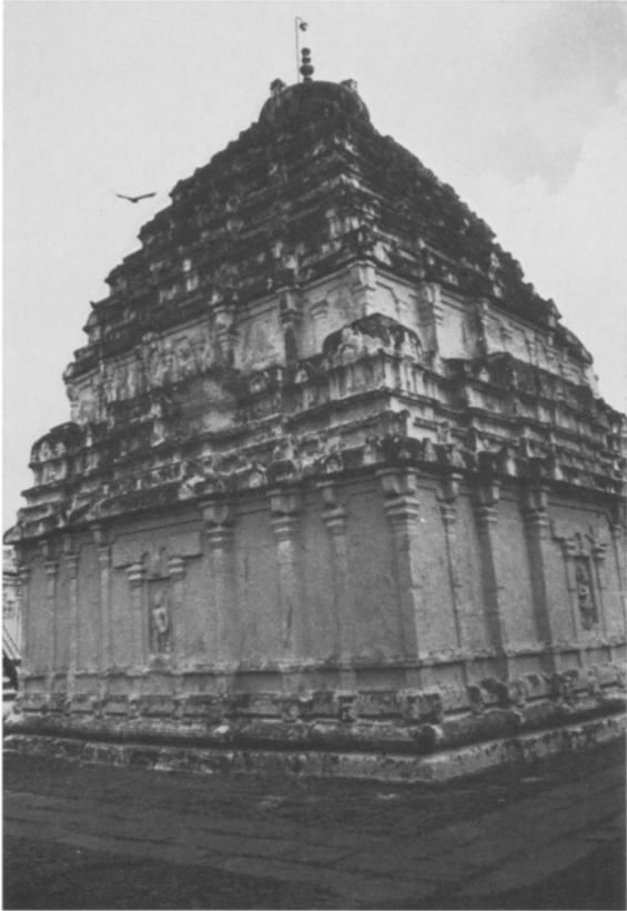
Fig. 15 Sandur, Pārvatī Temple, Bellary District, Karnataka, view from southwest
