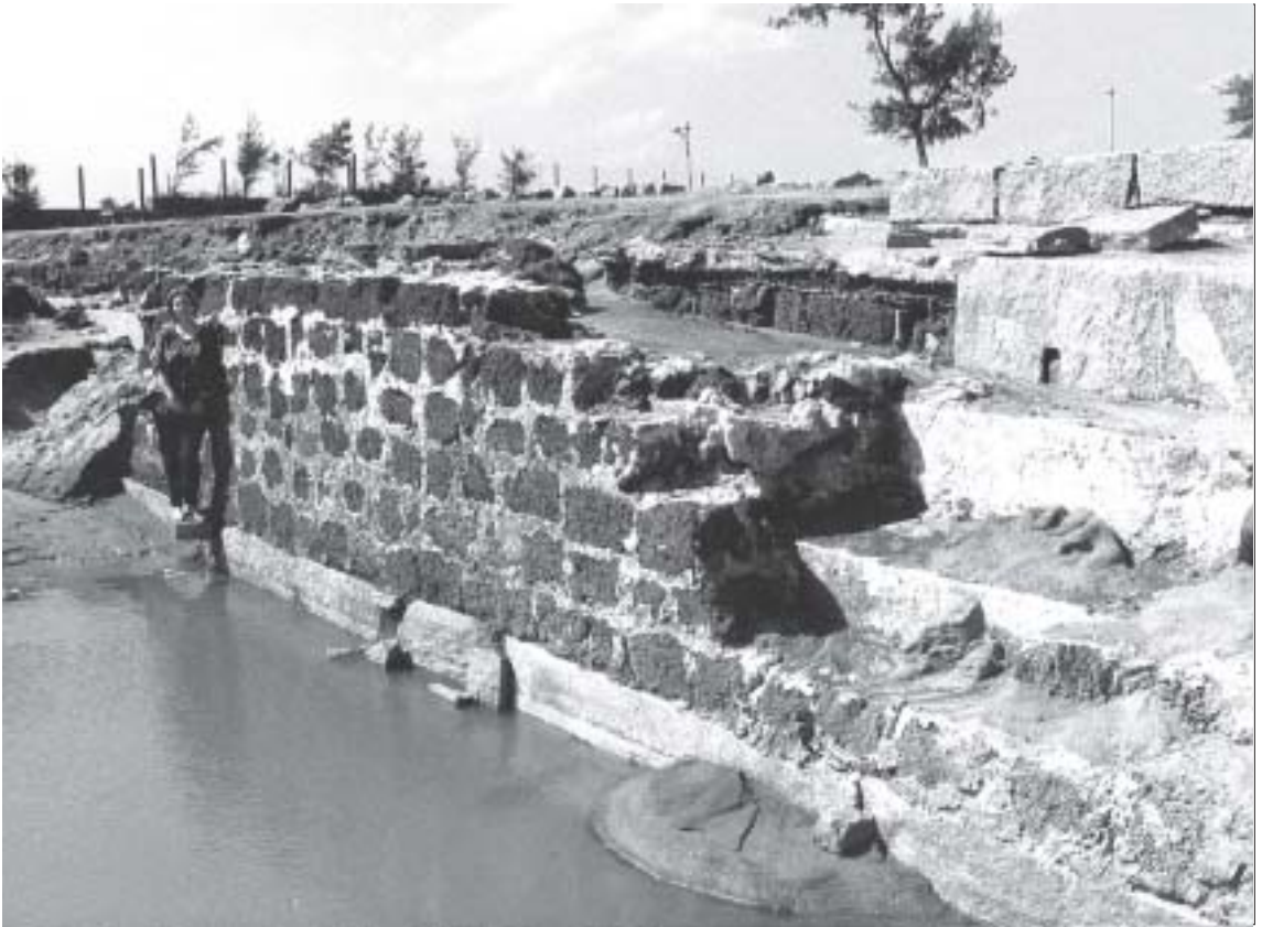
Breakwater wall – intact section
