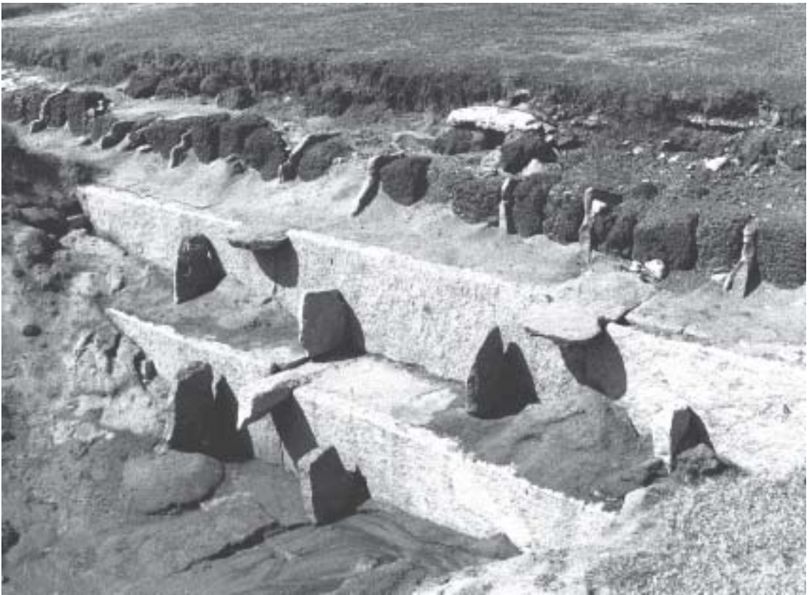
'Keyed' structure – Breakwater foundation
